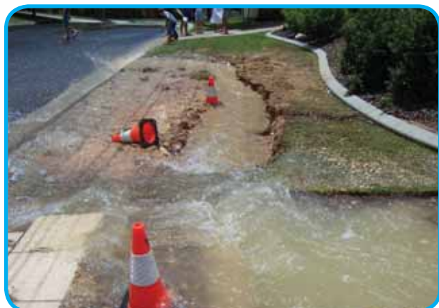
An example of high pressure causing a burst pipe and water wastage.
