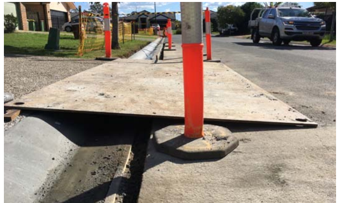
Typical access provided to driveways where kerb is being replaced.
