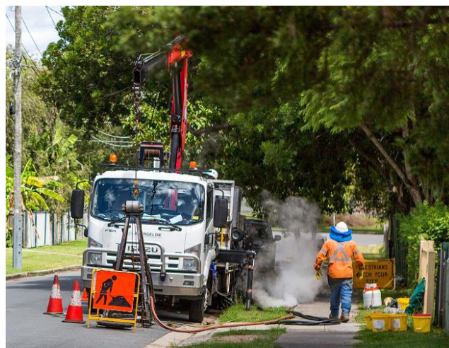
Pipeline relining in progress
