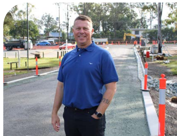
Cr Scott Bannan at Jimboomba Park during the reconstruction of the South Street driveway.
